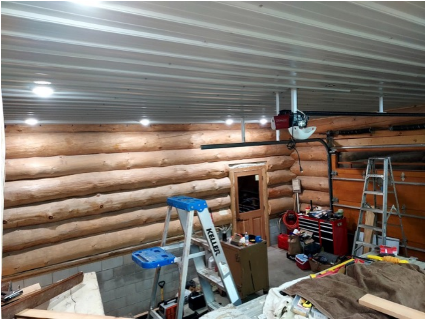
(Picture – Completed metal ceiling with custom brackets)
