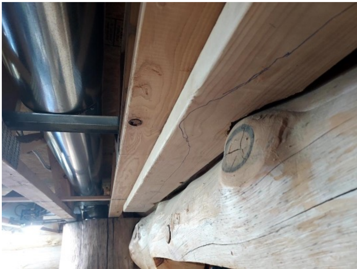
(Picture – Strong back & filler with the scribe line made with a wood shim scribe.)
